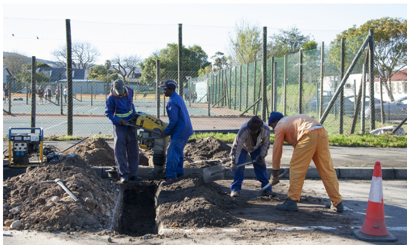
Reticulation Servicemen laying pipes in Knysna, RSA ©Outcomes Publishing
